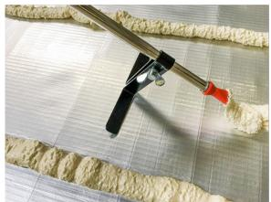
7. Apply the appropriate amount of SikaRoof® Board Adhesive according to the roof wind-load zone requirements.
