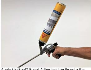
6. Apply SikaRoof® Board Adhesive directly onto the surface, then quickly press the insulation panel onto the flat roof with light pressure and adjust. Use the spacer to ensure right distance between the nozzle and a substrate.
