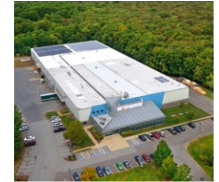
ENERGY SAVING PROGRAM AND SOLAR ENERGY SOURCING, SIKA CORPORATION PLANT CANTON, USA
