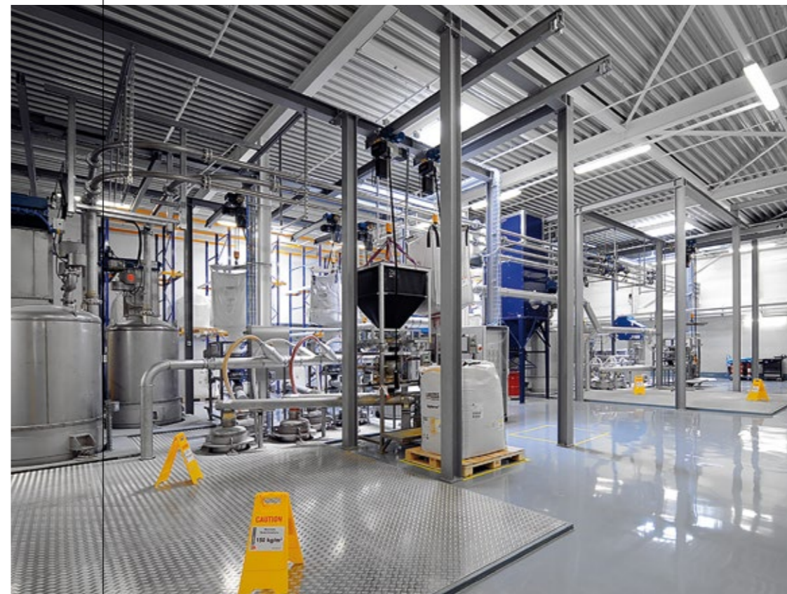
RECOVERING WASTE HEAT, SIKA MANUFACTURING PLANT DUEDINGEN, SWITZERLAND
