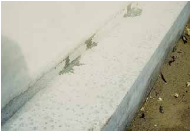
Simple injection process on site
