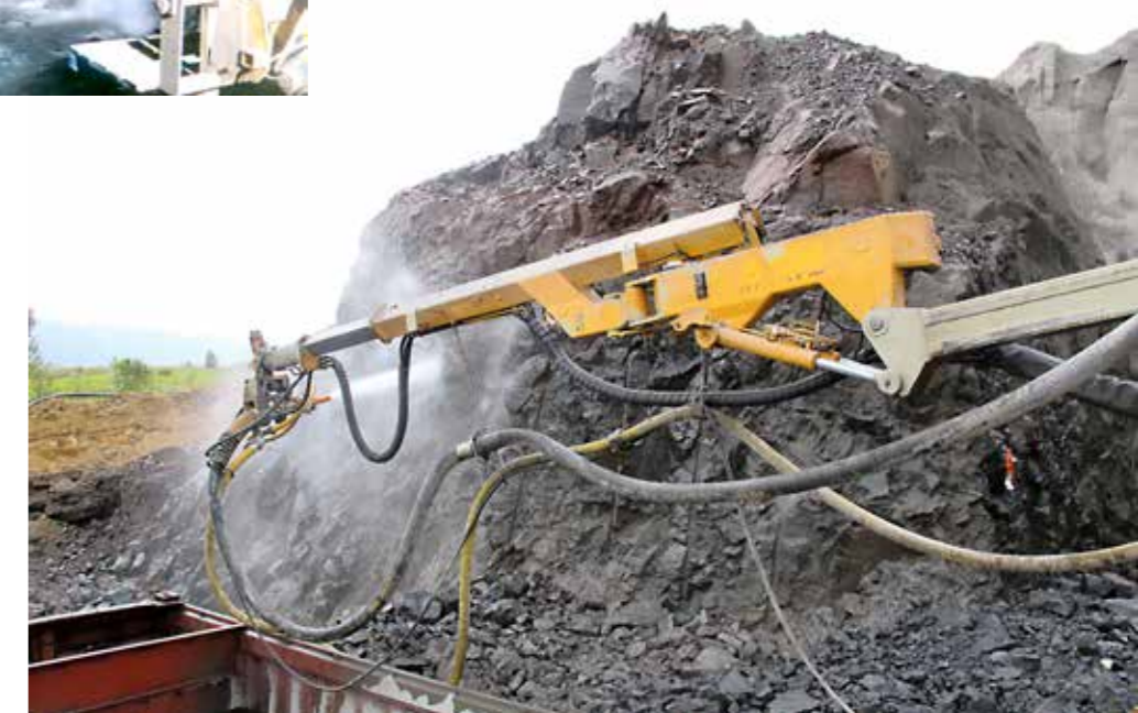
Testing the shotcrete, modified with Sika technology, for the right properties.
