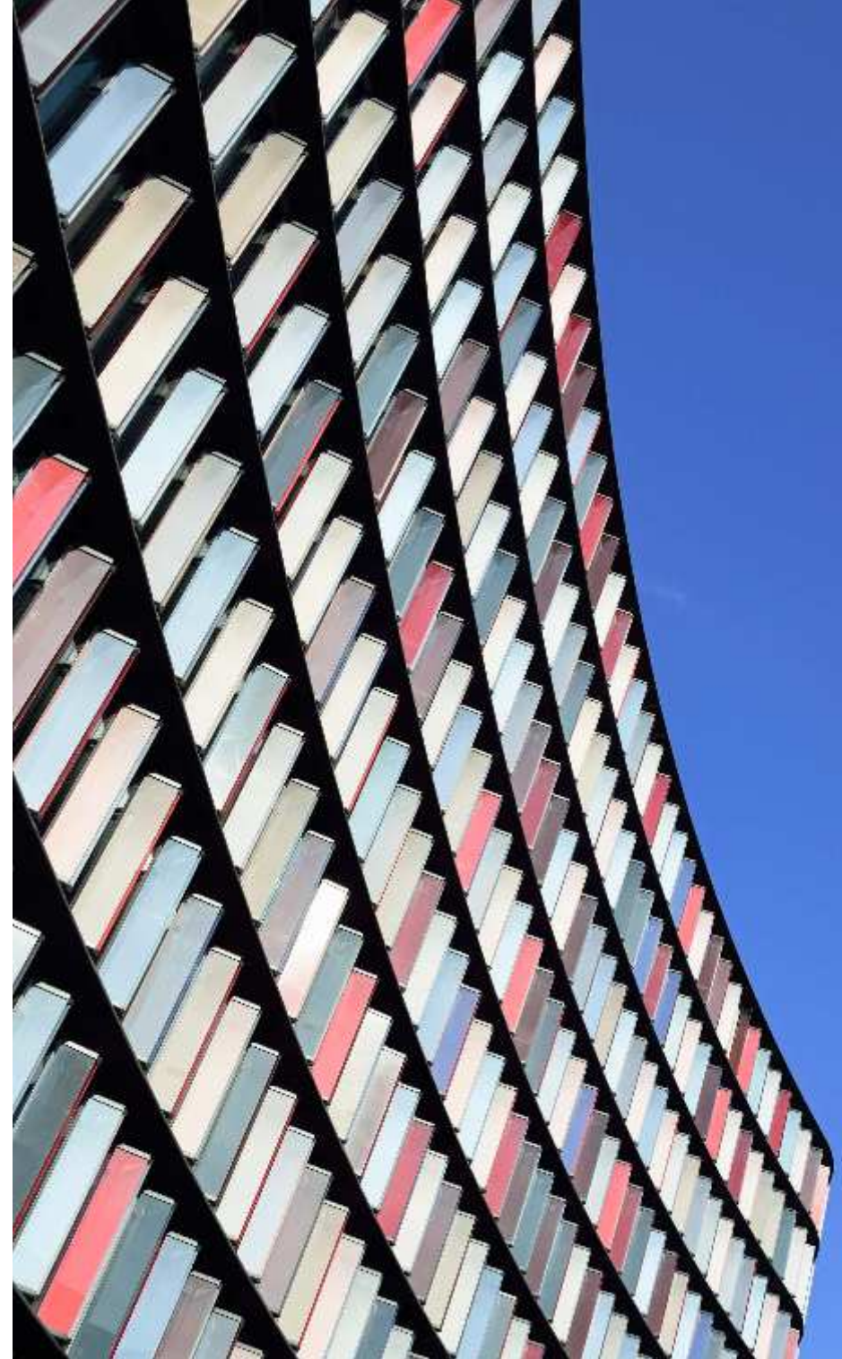
RIGHT, Project 80: Two New Ludgate Project Participants Architect: Sauerbruch Hutton Facade: Josef Gartner (2015)
