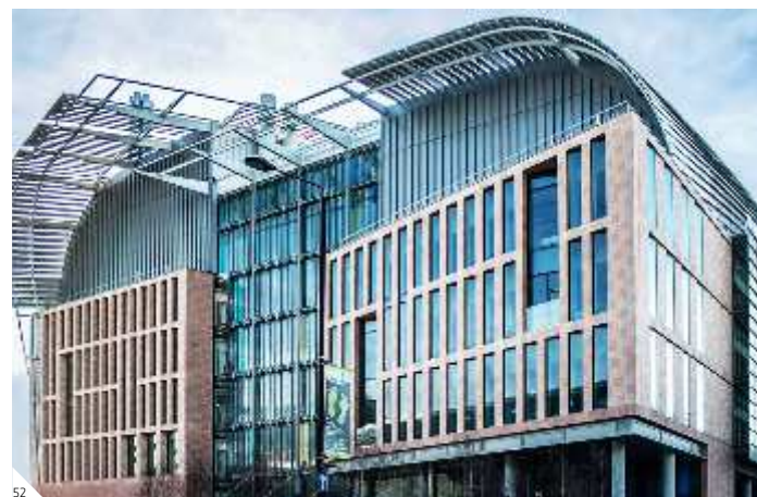
Francis Crick Institute Architect: HOK, PLP Architecture Facade: Scheldebouw, Josef Gartner (2016)
