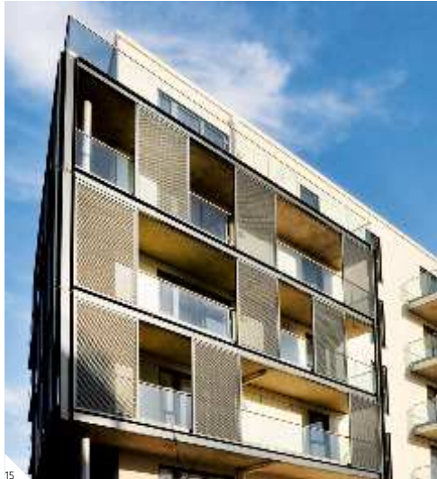
Threshold Residence, Parsons Green Project Participants Client: Threshold Housing Association Facade: Cladding UK
