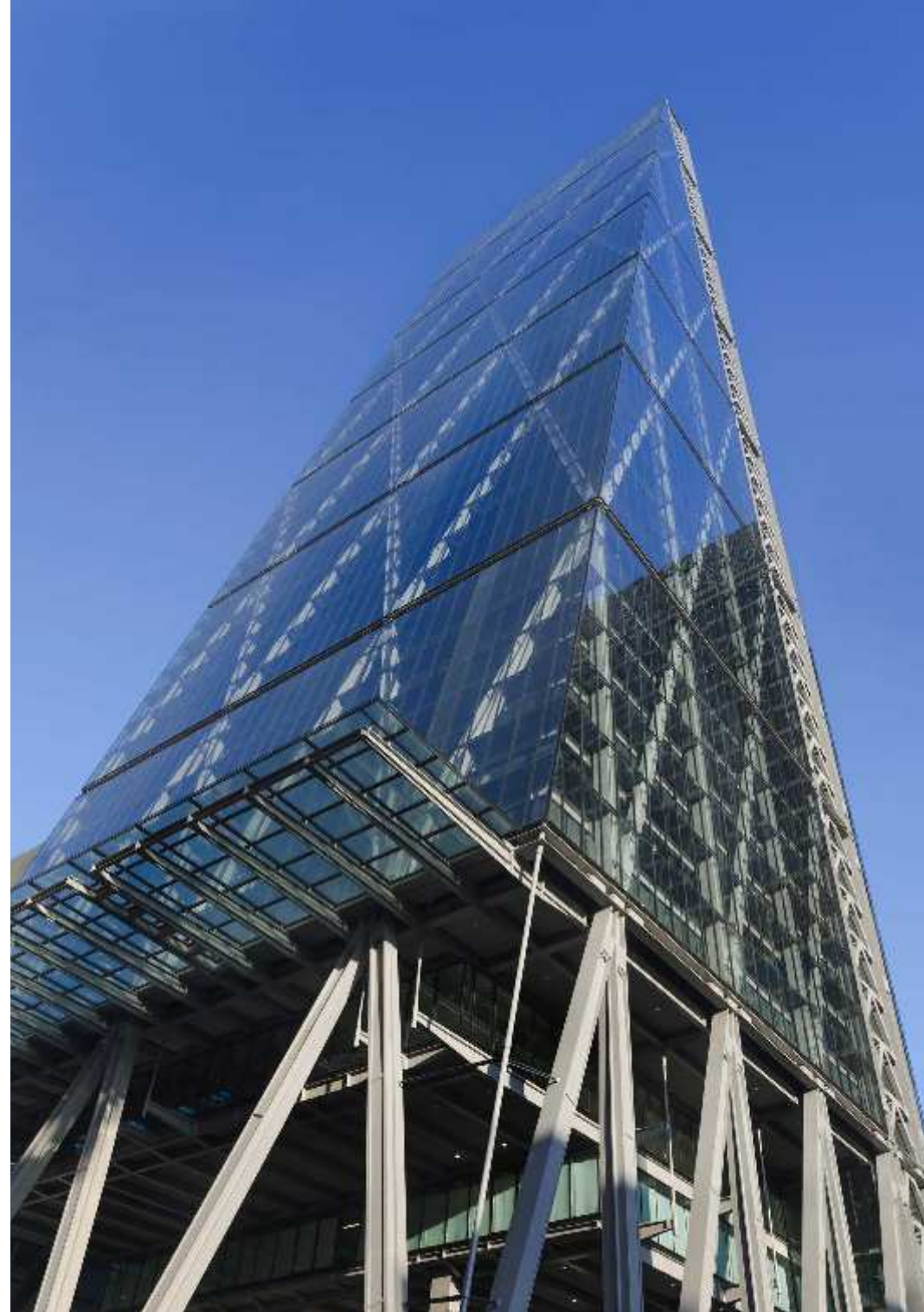
RIGHT, Project 114: 122 Leadenhall Street Project Participants Architect: Rogers Stirk Harbour + Partners Facade: YuanDa (CN) (2013)
