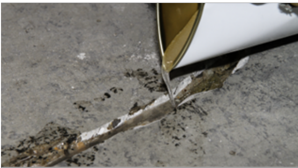
Pouring SikalInject®-1360 directly into the V-shaped groove opened on the crack
