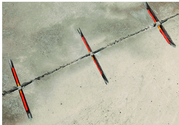
Placing the screed ties into the canals opened on the cracks
