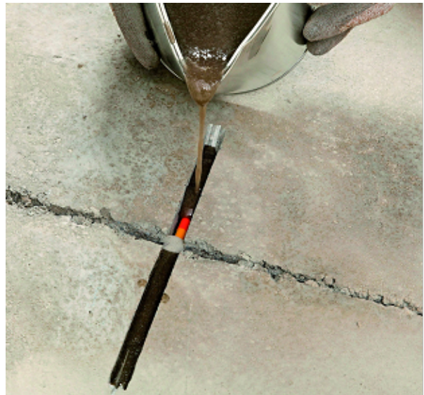
Filling the screed tie canals and crack with SikalInject®-1360 mixture.
