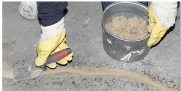
Levelling the crack surface by using proper Sikadur® / Sika MonoTop® mortar.
