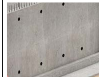
SikaSwell® Rings and Plugs Sikadur® 31 Sealing tie bar holes
