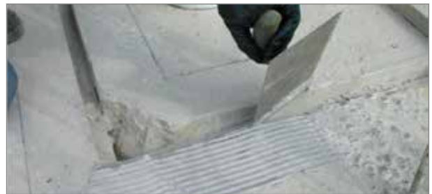
■ 2. Applying the base layer of adhesive
