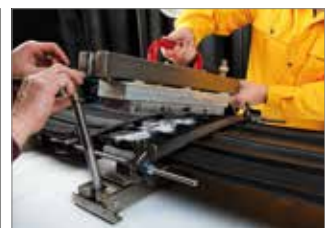
Powdering of waterstop and inserting into the vulcanizing equipment
