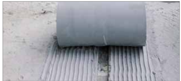
■ 3. Positioning the membrane strip
