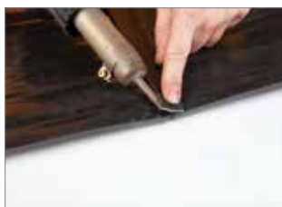
Strengthening with welding foil using hot air gun
