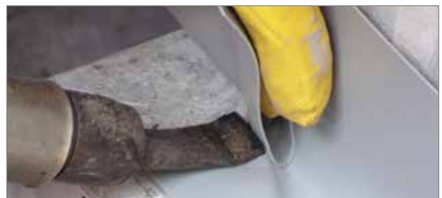
■ 4. Jointing membrane strips by heat welding
