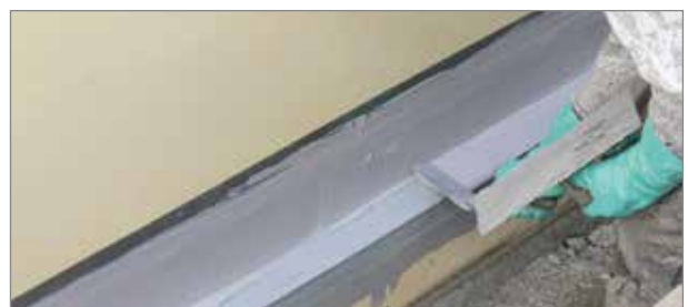
■ 5. Applying the top layer of adhesive
