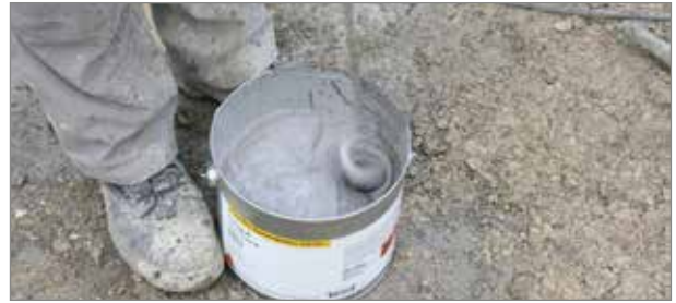
■ 1. Mixing the Sika® Tricoflex® FU 60 system adhesive
