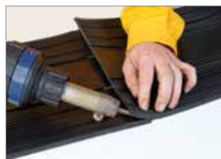
Overlapping joint with hotair blower
