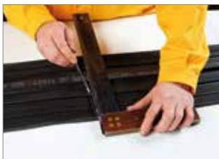
Measuring, marking, cutting
