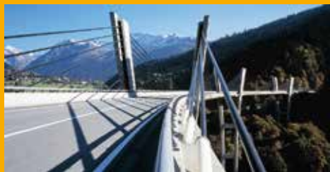
CONCRETE REPAIR AND PROTECTION
