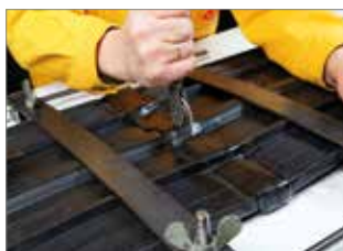
Application of cover strips; pressing home of both cover strips
