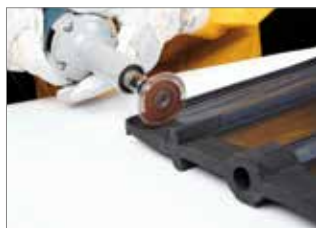
Grinding of the rubber surface
