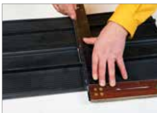
Measuring, marking, cutting
