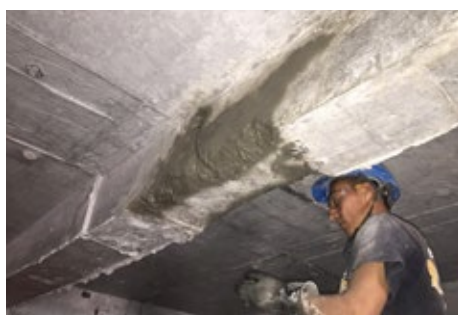
Concrete repair and refurbishment, Page 28
